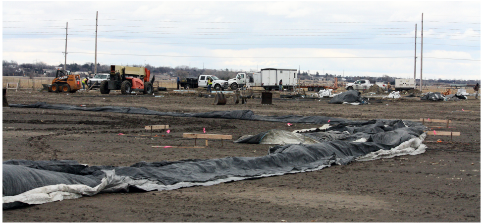
STILL WORKING - Work continues on the new high school.
